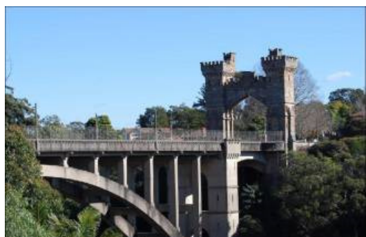
FENCED IN: The RTA's chosen design for the safety fence at Long Gully Bridge.
